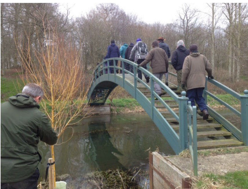
The bridge at St Helen's
